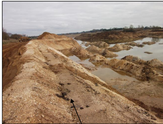
Photograph 3: Existing slope into current extraction area
